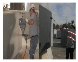
IMRAE **CoatMasters® 7007** Dampproof and Waterproof Coating can be easily applied, by either roller or spray, for quick set-up and clean-up operation.
